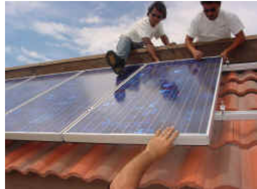
The Tile Trac® with a tile roof. Photo courtesy of Advanced Solar Electric
