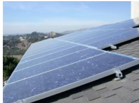
The Tile Trac® keeps a low 3" profile to composition roof-tops.
